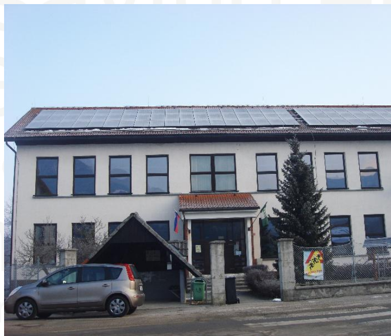
Solar system on the school building.
