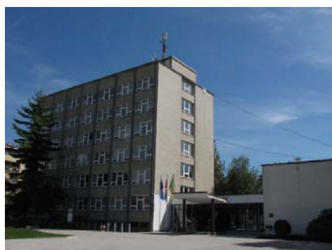
Municipal Building of the Municipality of Velenje
